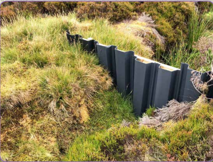
Drainage channels dug in the 1960s have led to the drying out of peatland
